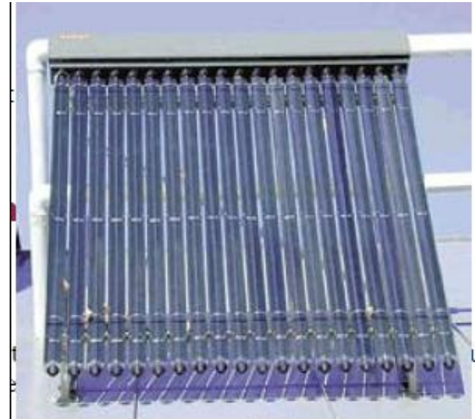
Figure 6.18 An evacuated tube collector re collector (see Figures 6.16 and 6.17)
