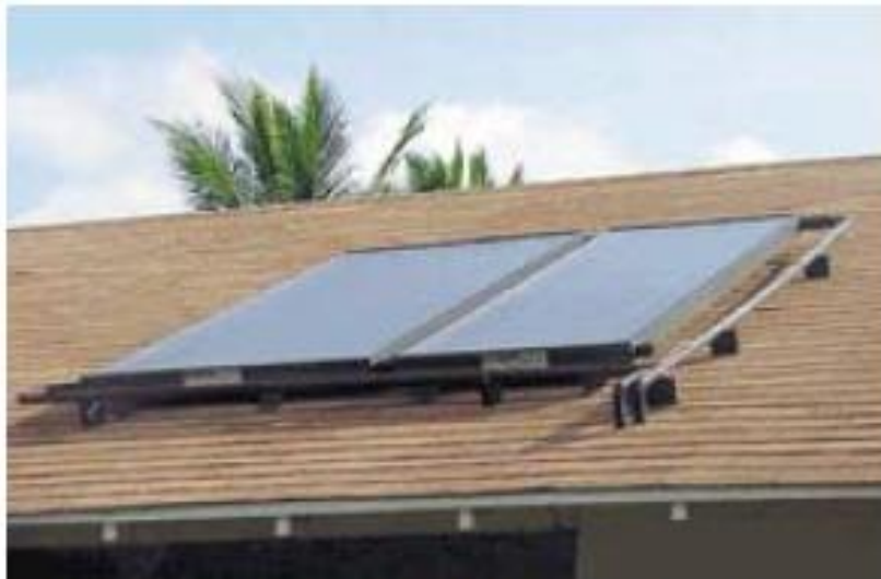
Figure 6.16 Solar flat collectors on a roof.
